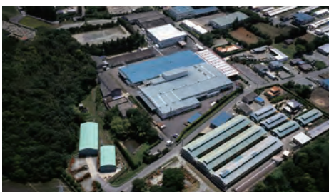
● 三重工場 Mie Plant Site: 42,259 m 2 (454,872 sq.ft.) / Floor space: 25,405 m 2 (273,457 sq.ft.)
