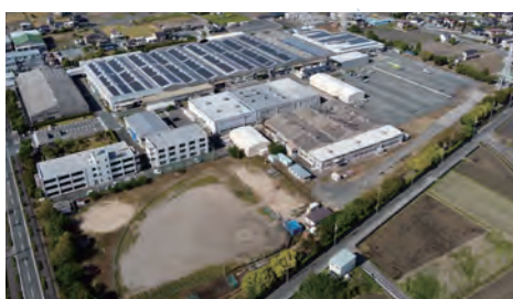
● THKリズム (株) 本社・浜松工場 THK RHYTHM CO., LTD., Headquarters and Hamamatsu Plant Site: 97,629 m 2 (1,050,870 sq.ft.) / Floor space: 43,485 m 2 (468,069 sq.ft.)
