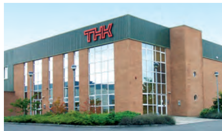
● THK Manufacturing of Ireland Ltd. (Ireland) Site: 10,198 m 2 (109,771 sq.ft.) / Floor space: 4,291 m 2 (46,188 sq.ft.)
