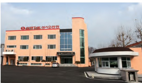
● SAMICK THK CO., LTD. Seongseo 2 Plant (South Korea) Site: 10,119 m 2 (108,920 sq.ft.) / Floor space: 6,874 m 2 (73,991 sq.ft.)
