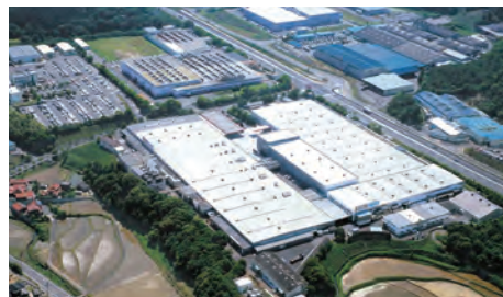
● 山口工場 Yamaguchi Plant Site: 160,798 m 2 (1,730,818 sq.ft.) / Floor space: 77,912 m 2 (838,641 sq.ft.)
